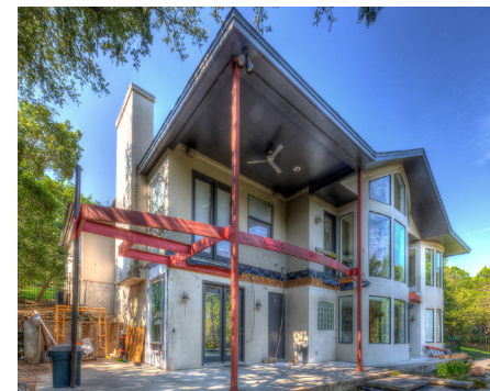
Terrace Under Construction
